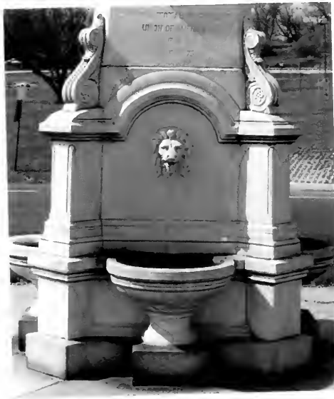
Figure 34: Stain on pedestal under lion head spout (Photograph by author, March 2002)
